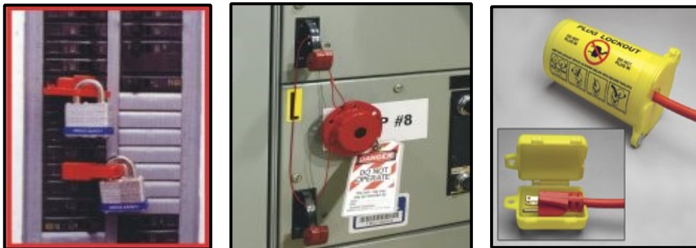
Locks and Tags on Single and Multiple Electrical Breakers Electrical Plug Lock Box
