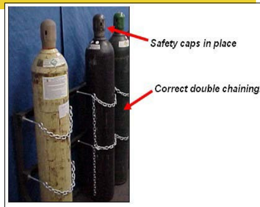
Figure 8.3 – Cylinders Stored and Chained Correctly
